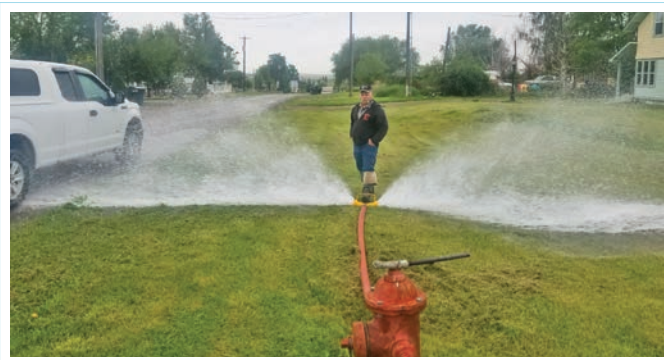
Jeff Cook helps sanitize and flush the system in Dietrich Idaho after a system malfunction.
