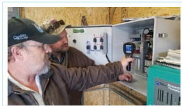
Craig Sturman, Circuit Rider, assisting the City of Ucon diagnose an electrical problem at a lift station using a FLIR (forward looking infrared radar).
